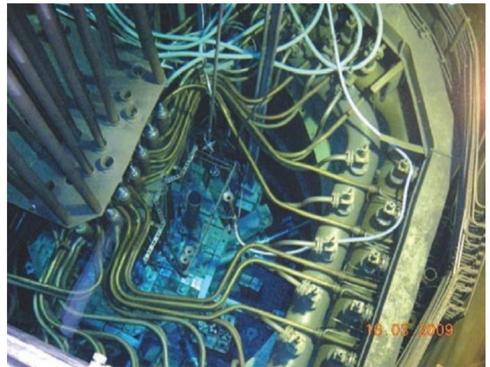
**The MARIA research reactor operated in National Centre for Nuclear Research (NCBJ) in Świerk. Light blue glow seen deep inside the reactor core is the Cherenkov radiation**
